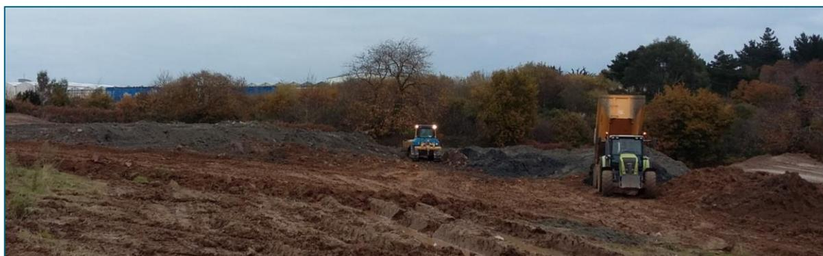
FIGURE 44 – CREATION D'UNE PLATE-FORME MARAICHERE, A L'AIDE DE SEDIMENT, DESTINEE A ACCUEILLIR DES SERRES (PAIMPOL, 2015)
