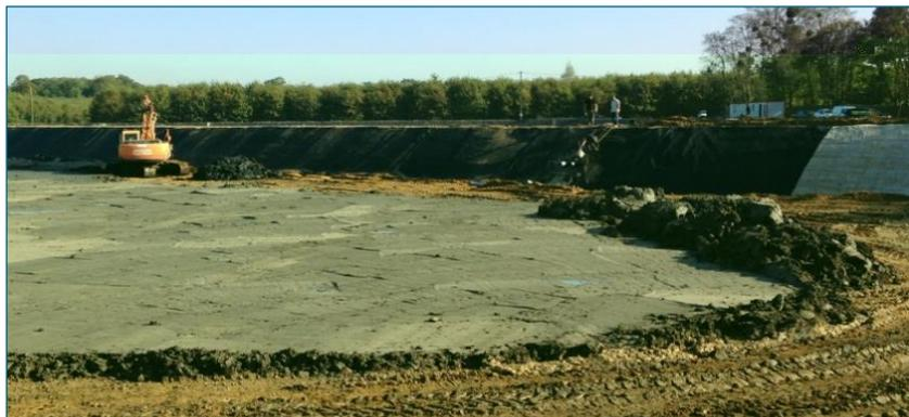
FIGURE 55 – MISE EN ŒUVRE D'UNE BARRIERE PASSIVE (LA HISSE / IDRA, 2018)
