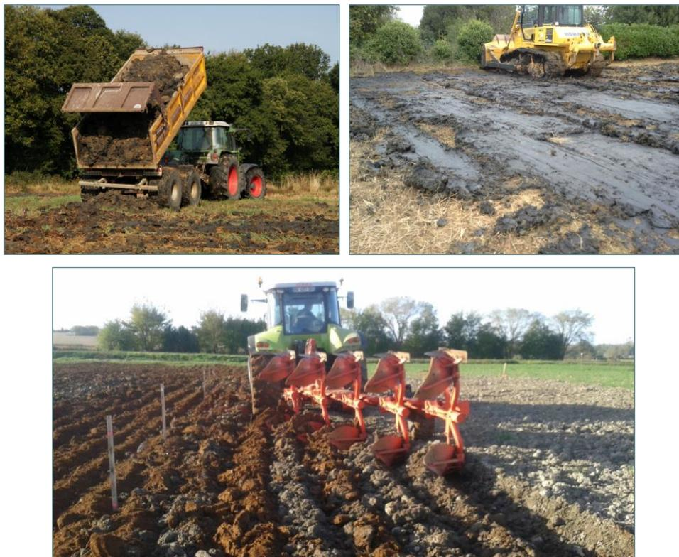
FIGURE 40 – EPANDAGE DE SEDIMENT (COEUR E. / IDRA, 2018 ; CA 17)
