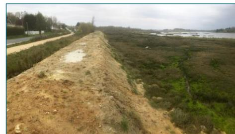
**FIGURE 43 – DIGUE SECONDAIRE DE PROTECTION CONTRE LES SUBMERSIONS (IDRA, COMMUNE DE SENE, 2018)**
